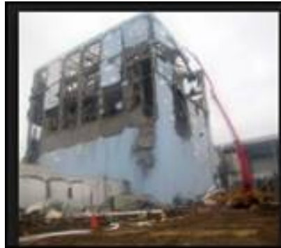
Fukushima Daiichi, Unit 4- Hose adding water to pool, reactor building is a shell after explosion
